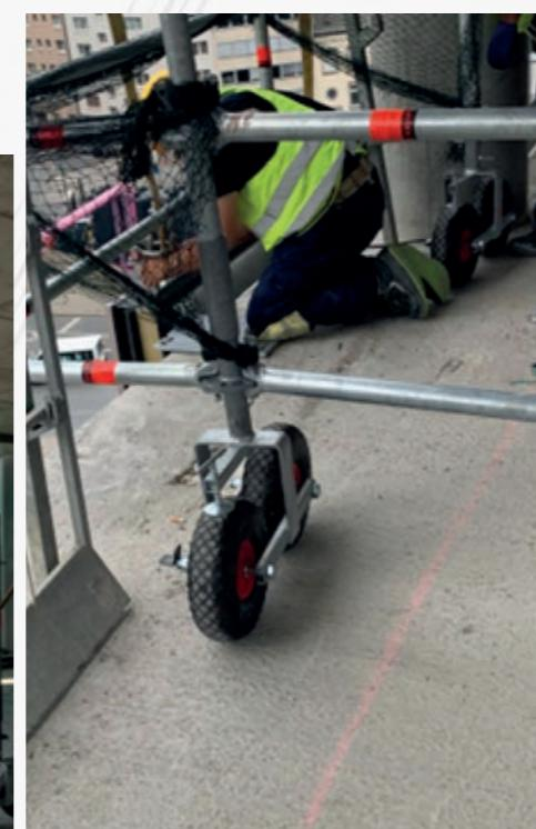
Bracket installation on the floor involves checking holes drilled on concrete slabs, marking anchor points on steel, installing appropriate anchors based on shop drawings, ensuring proper position, and fixing with nuts and bolts using torque keys.
